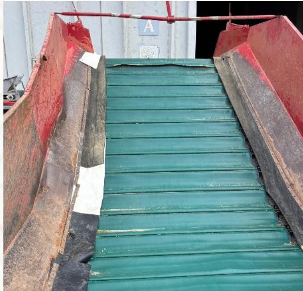
Figure 2. Sealing Improvement Applied to Elevator Surface
